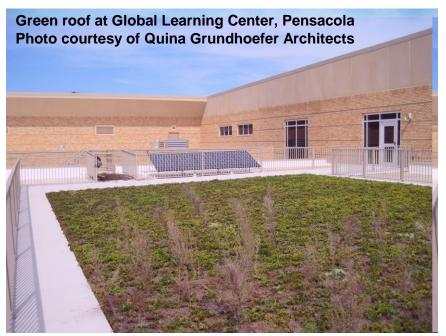
collected in a cistern or, if the greenroof is part of a BMP Treatment Train, the filtrate may be discharged to a downstream BMP such as a wet detention pond. A cistern is sized for a specific amount of filtrate and receives no other stormwater. Other pond storage must also provide capacity to detain a specified quantity of filtrate.
