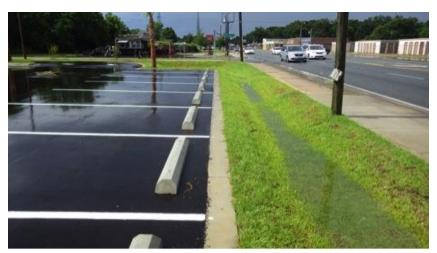
locations. Pavement must be graded so that stormwater flows through the curb cuts onto the vegetated area. Thus, roadways and other paved areas can be changed from DCIA to non-DCIA areas, reducing the calculated required treatment volume.
